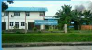
Bio-Mass Power Plant 15 MVA
