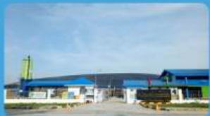
Bio-Gas Power Plant 10 MVA
